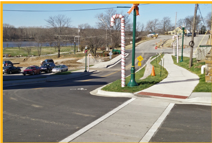
Crosswalk, bike lane, wide sidewalks and curb ramp.
