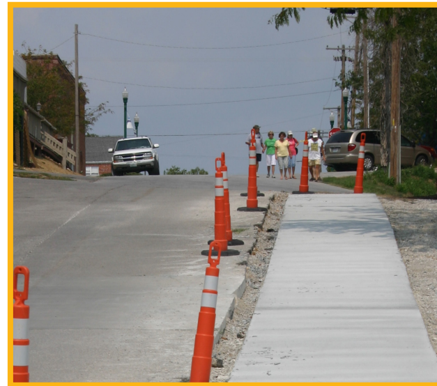
Sidewalk construction in Warsaw, Mo
