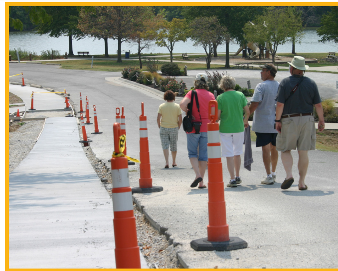
Warsaw, Mo sidewalk construction
